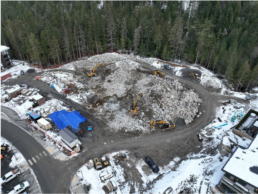
Lot 3 – Current Site Conditions
