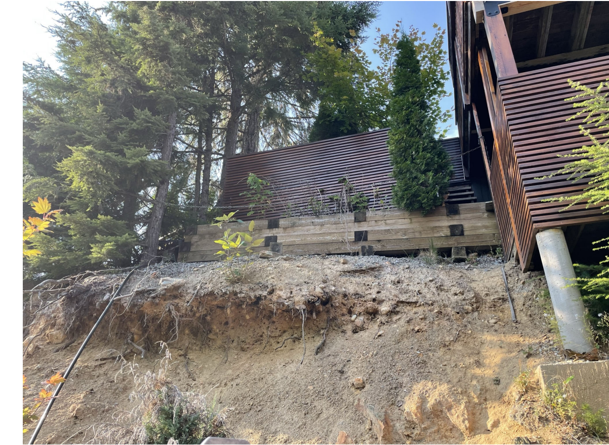
IMAGE OF ENCRDACHING POST & SLOPE
